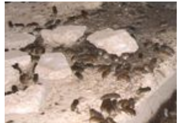
Rats can chew and tunnel through old crumbling cement.
